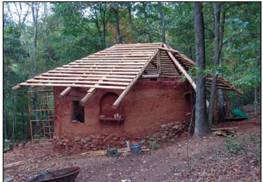
Views of the interior and the roof going up. The walls were built before the roof, but they wouldn't repeat that process again.
