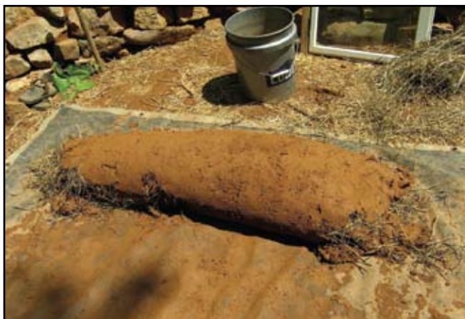
“Cob” is simply clay earth, sand, water, and straw. Views of the foundation-building in progress.
