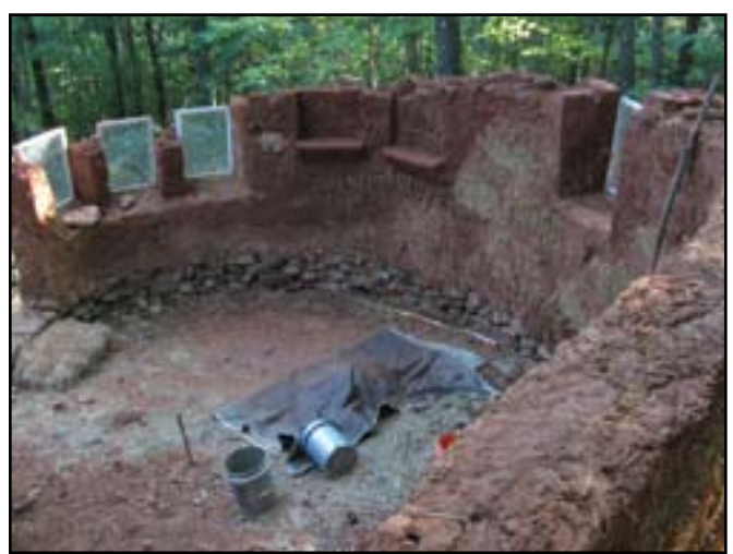
“Cob” is simply clay earth, sand, water, and straw. Views of the foundation-building in progress.
