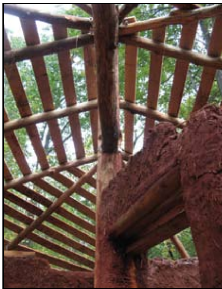
Views of the interior and the roof going up. The walls were built before the roof, but they wouldn't repeat that process again.
